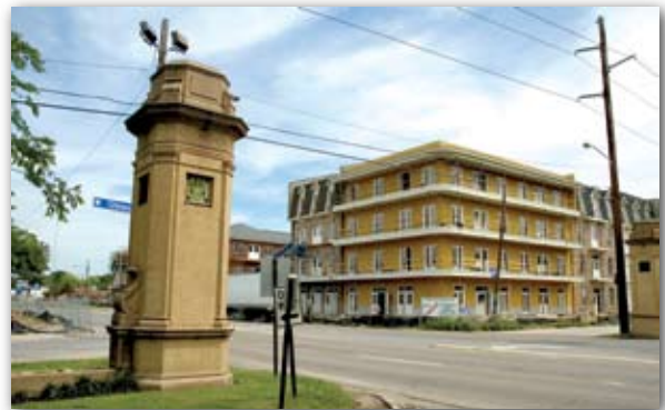
FieldHouse Sports Lofts are among hundreds of new units at LSU's North Gates
