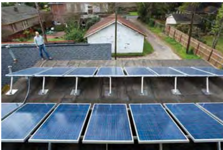
Adam Knapp inspects the solar panels, which will provide a return in four years or less.
