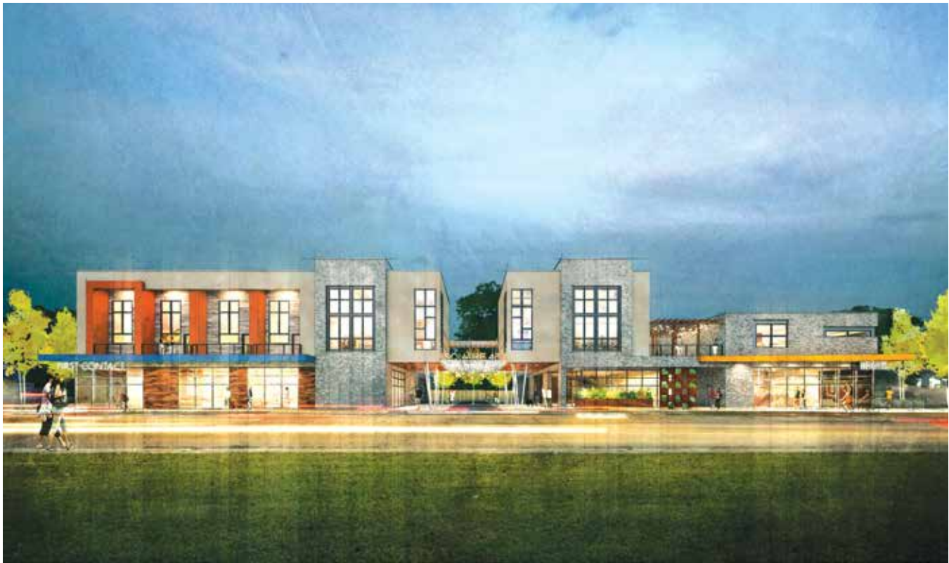
When Square 46 is completed this summer, it will have retail, apartments and the White Star Market, a number of small restaurants in the configuration of a food market. Square 46 is on Government near Foster Drive.
