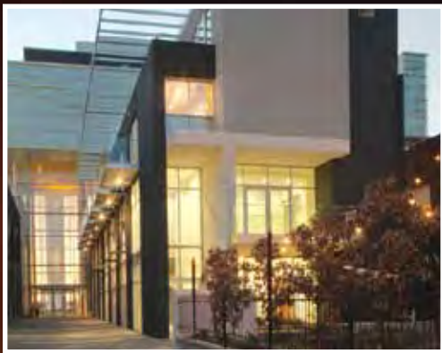
2008 —OneEleven Lofts open on Third Street in Downtown Baton Rouge.
