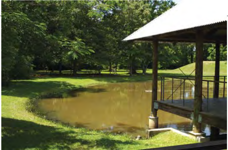
To the existing pavilion overlooking the pond, LSU's Hilltop Arboretum will add a building, bridges and more.
